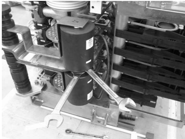
Figure 8-7 Loosening the Middle Connection
